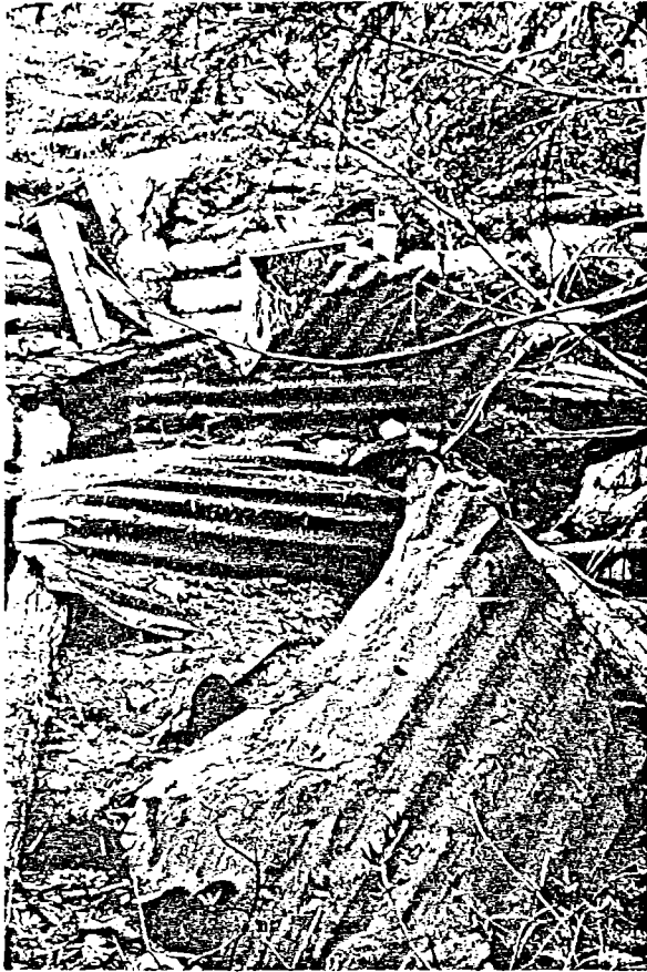
Brosius cabin. Corrugated metal roofing outside cabin near southwest corner, looking northeast.
