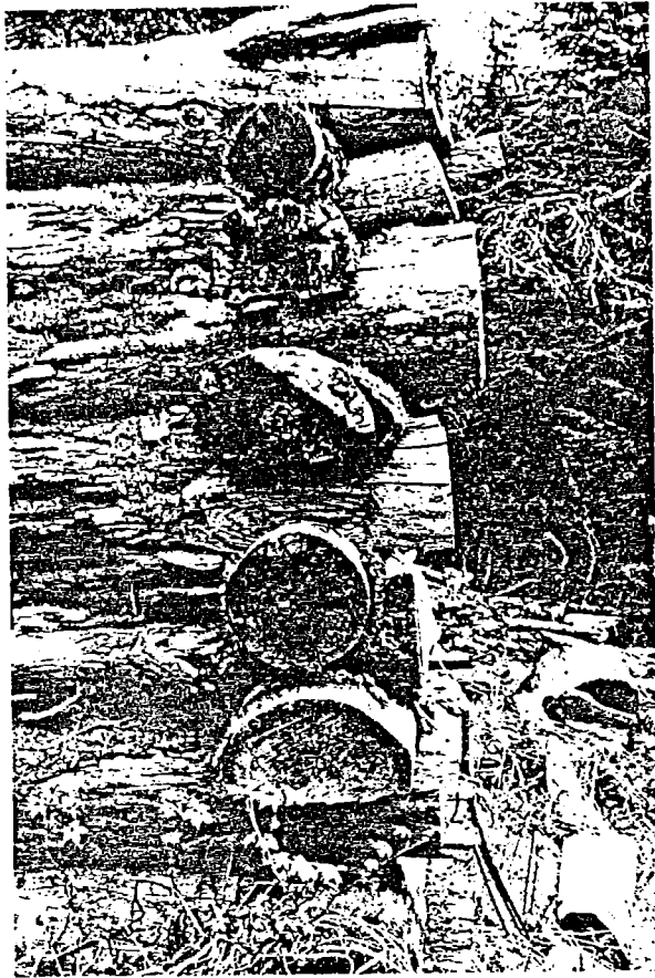
Brosius cabin. Detail of construction of northwest corner, looking south.
